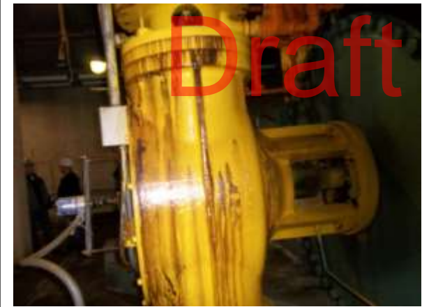
Oil hydraulic valve actuators leaking oil
