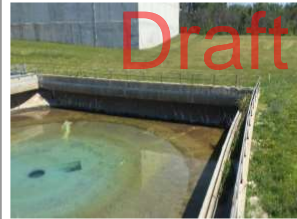
Raw sludge clarifier at Lake Huron WTP
