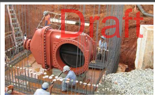
A large valve for a transmission pipe.
