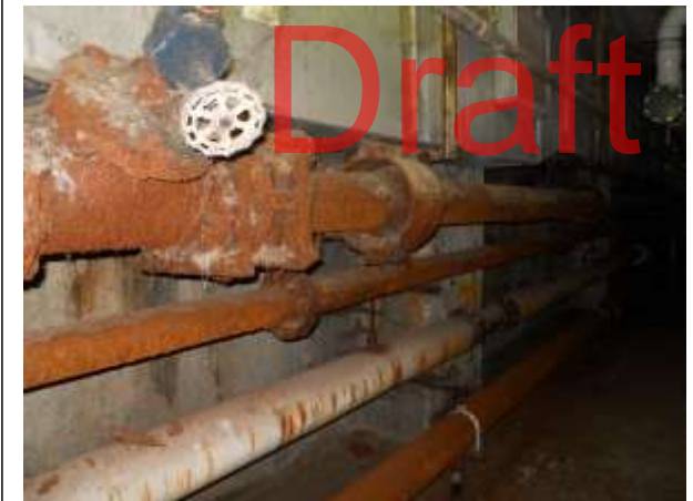
Multiple pipe lines such as Potable Water, Screened Final Effluent, Natural Gas, and Compressed Air Pipe lines at the WRRF are aging, getting corroded, leaking and failing at the WRRF
