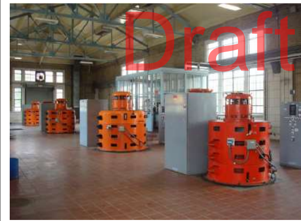
Sanitary pumps at Fairview Pumping Station
