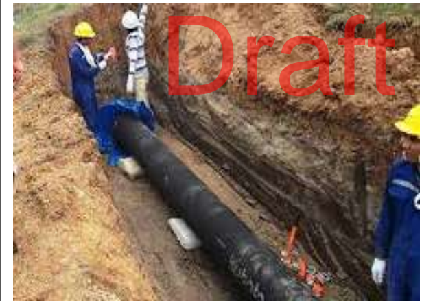
Water main being installed
