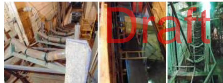
Picture from left to right Sludge Conveyor G Damaged by Fire and Conveyor B in the Complex – II Dewatering Building and Fire Damaged Conveyor H in Complex-II Incinerators Building.
