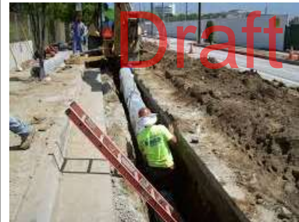
Water main being replaced
