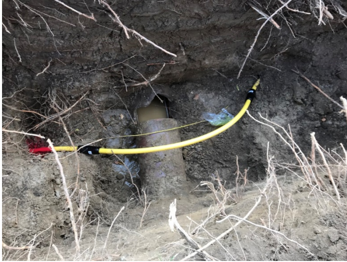
Repaired gas line. Sewer still needs to be repaired.
