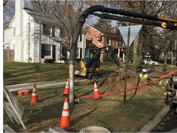
Working at cross-bore site. Orange line is jet cleaning line behind cross-bore
