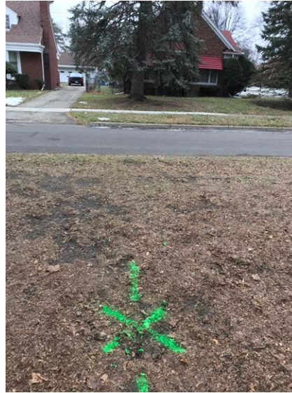
Marking Location of Cross Bore
