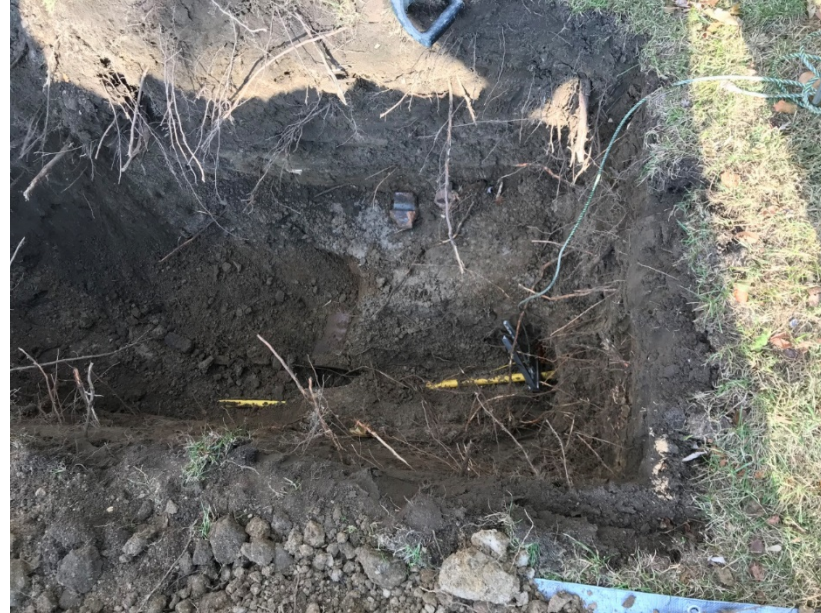
Excavated gas and sewer lines
