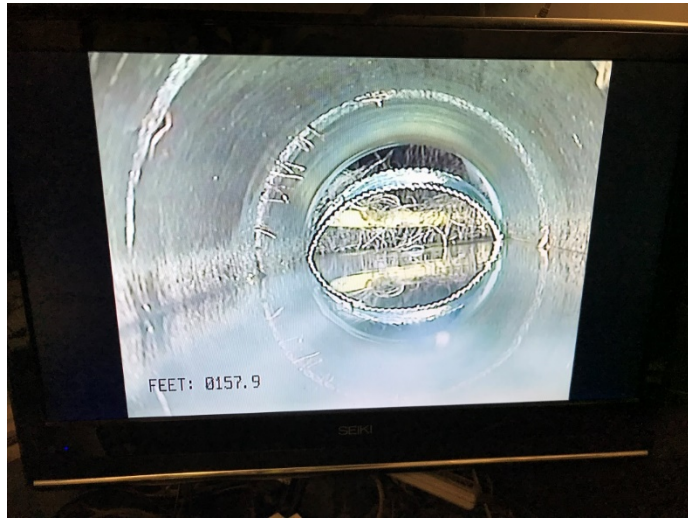
Cross-bore with roots and cutter
