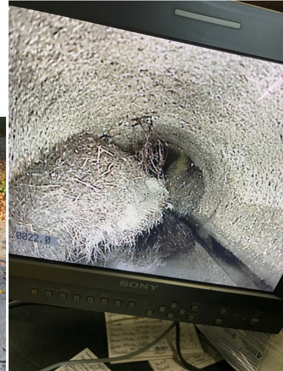
Root balls found in lateral, very common in abandoned house lots
