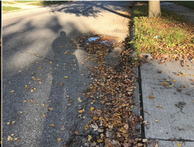
Pavement depression at collapse site
