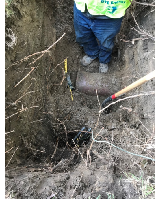
Excavated Cross-bore and cutter
