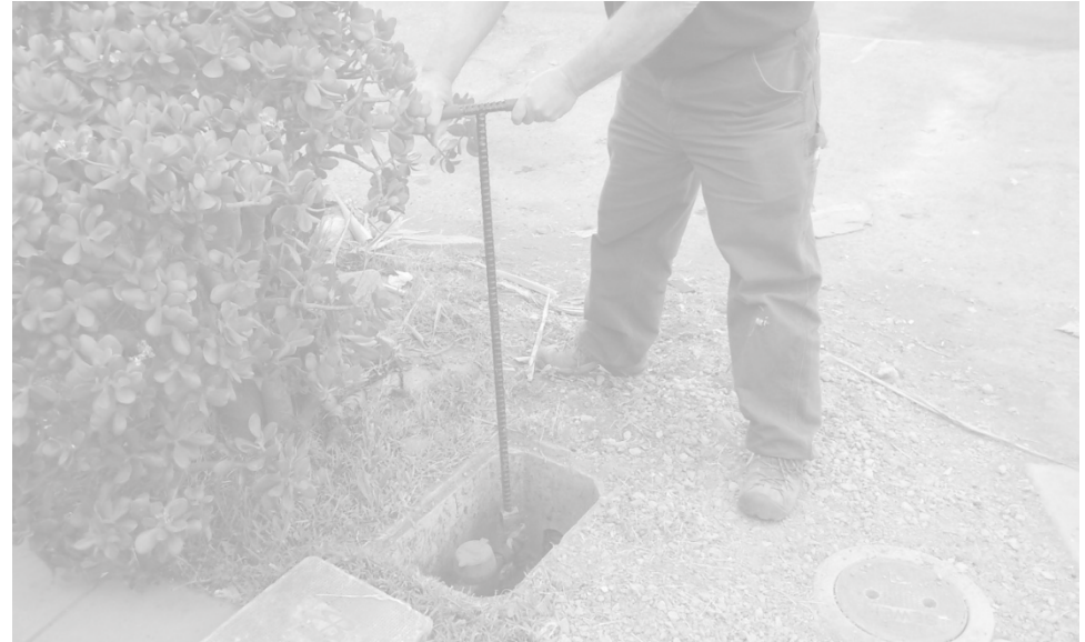
Water theft with unauthorized turn-on
