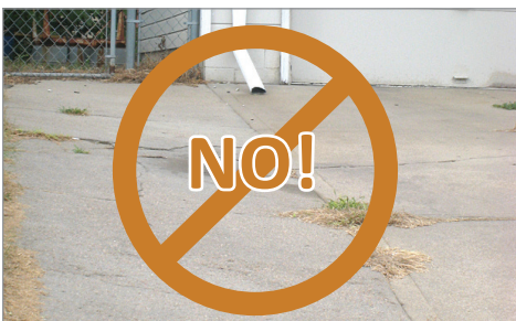
Downspout should not be directed to impervious areas as depicted in this example. Here stormwater flows down the driveway to the street. The discharge can also cause an icing hazard.
